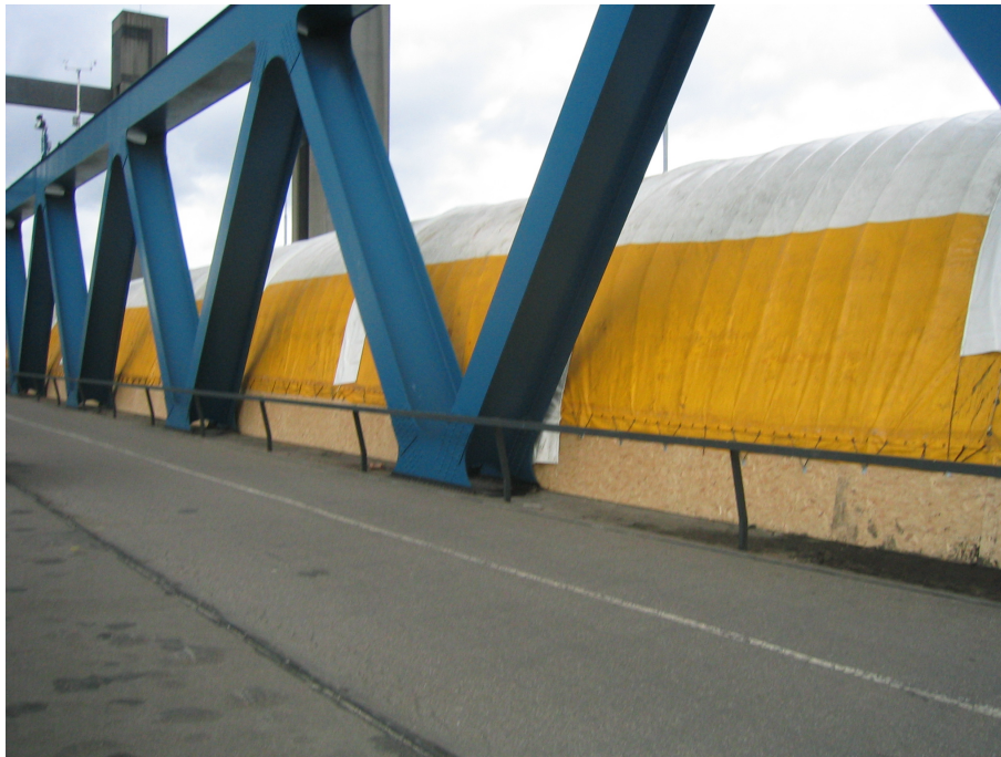
Fig. 6. Repairing a bridge deck with a fiber reinforced concrete C130, aiming at both durability and avoidance of further fatigue cracking.
