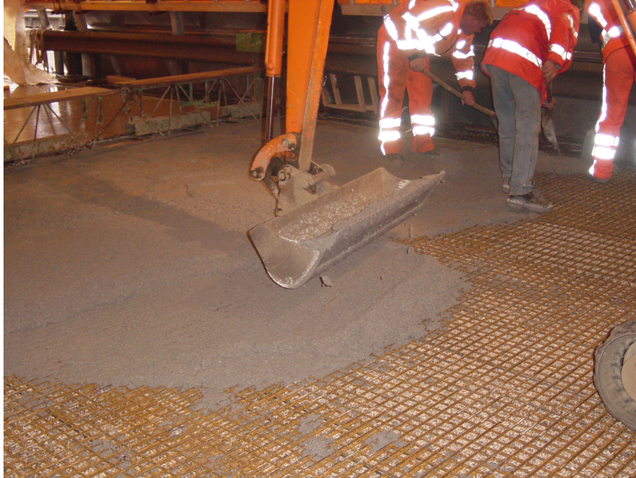
Fig. 3. Casting a high performance concrete bridge deck for bridge renovation in the Netherlands.
