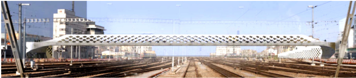
Negrellisteg, Zürich – Projekt/projet: Flint & Neill Ltd Civil Engineers, London; Explorations Architecture, Paris
